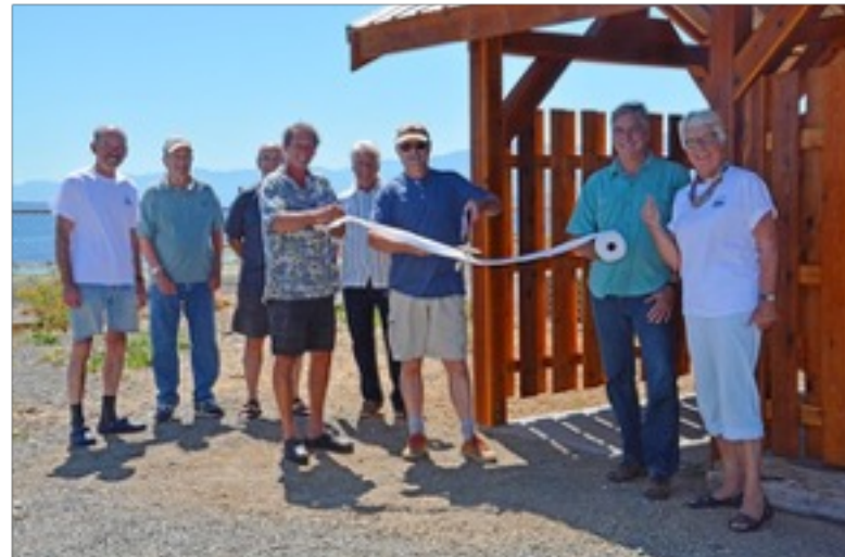
As volunteer stewards of their local beach, these residents of Comox, British Columbia designed and built this attractive structure that encloses a commercial porta potty.
