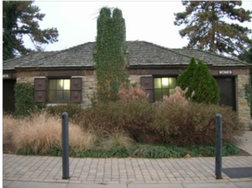
This comfort station in a Cincinnati park is typical of facilities built in the first half of the 20th century.
